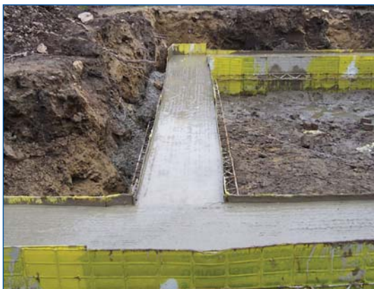
450mm x 450mm ground beams installed within Pecalif Shuttering System.
