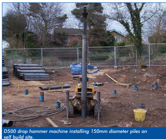
D500 drop hammer machine installing 150mm diameter piles on self build site.
