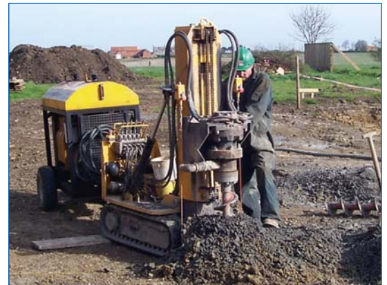
200mm augered piles installed with full heave precautions.
