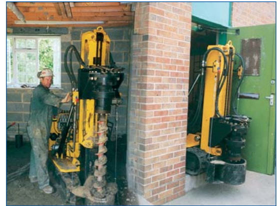
Auger rig with limited headroom/access situation.
