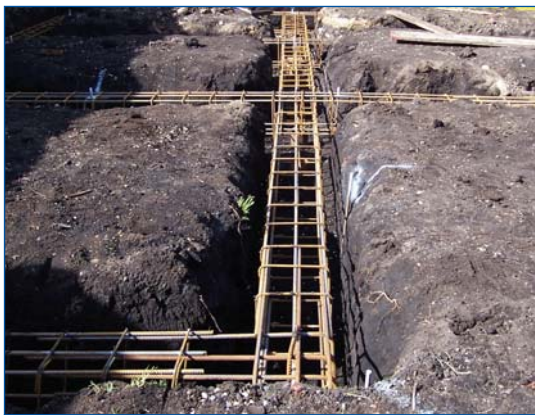
150mm steel cased piles and reinforcement within excavated trench, awaiting concrete placement.
