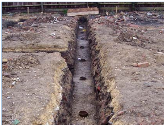
150mm steel cased piles awaiting ground beam construction.
